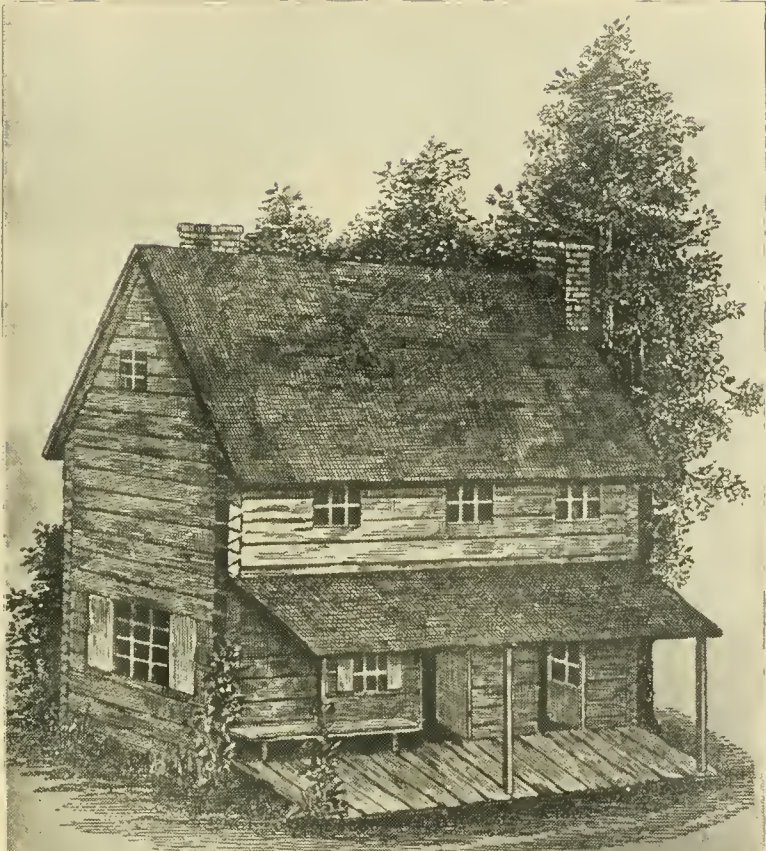
COLONEL'S QUARTERS, Fort Augusta. The above building stood inside of the Fort.
