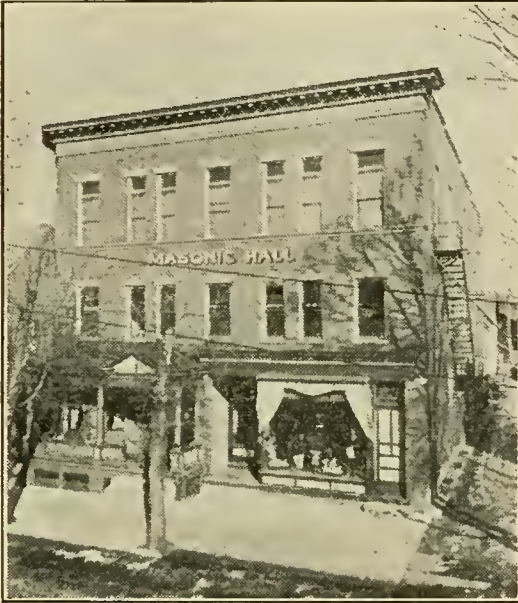
Present home of Watsonstown Lodge, No. 401.
